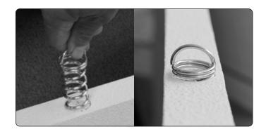
To install the Corkscrew, first carefully center the Corkscrew on the edge of the panel. Twist and push the anchor into the edge until it breaks through the coating and is flush with the panel. Be sure to keep the anchor as straight as possible and proceed slowly to avoid pushing through the face of the panel.
