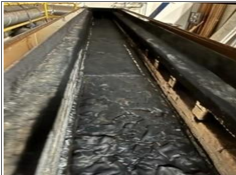
Photo No. 2 Post Test
