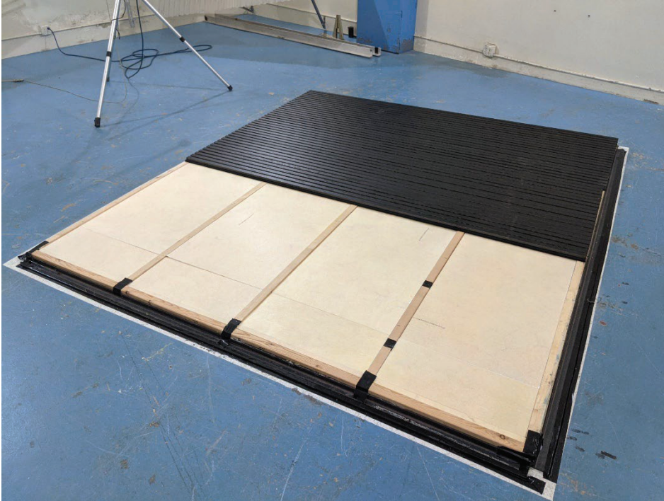
Figure 3 – ECOScapes panels partially installed over wood furring and glass wool
