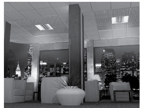
Radiator diffusers surround light fixtures in a hotel lobby ceiling.
